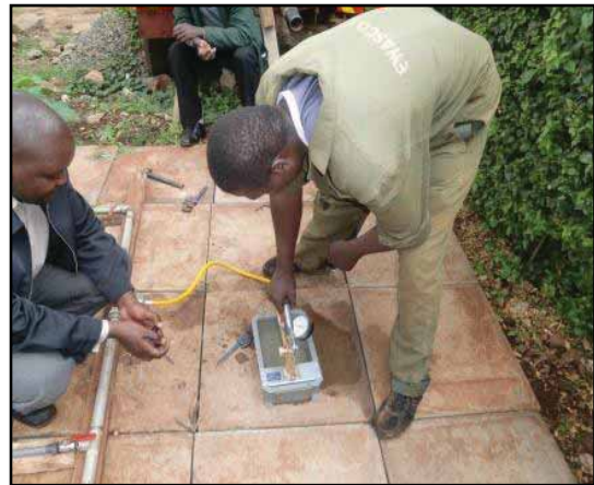
Connect pump with pipe and place water pressure gauge
